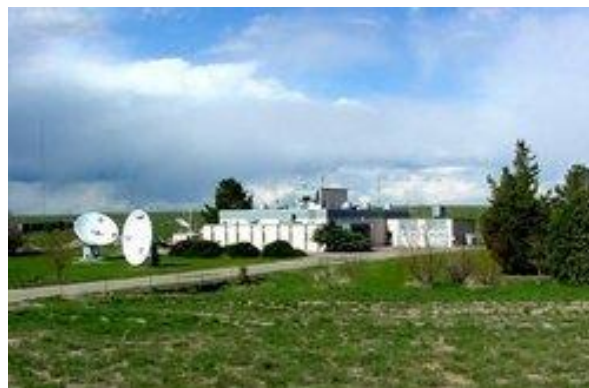
The WWV complex in Fort Collins, Colorado. [NIST photo]
